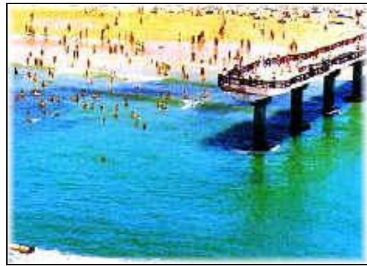
Figure 2.7: Hobie Beach pier
