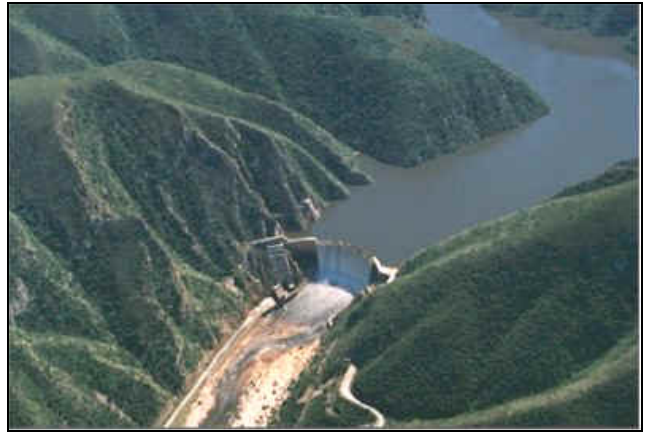
Figure 4.11: Kouga Dam on the Kouga River
