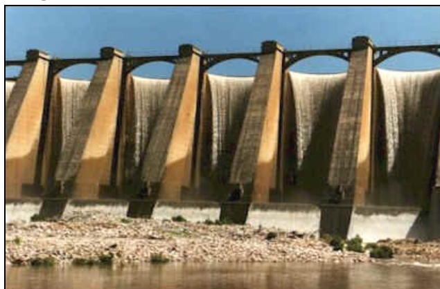
Figure 4.7: Churchill Dam wall
